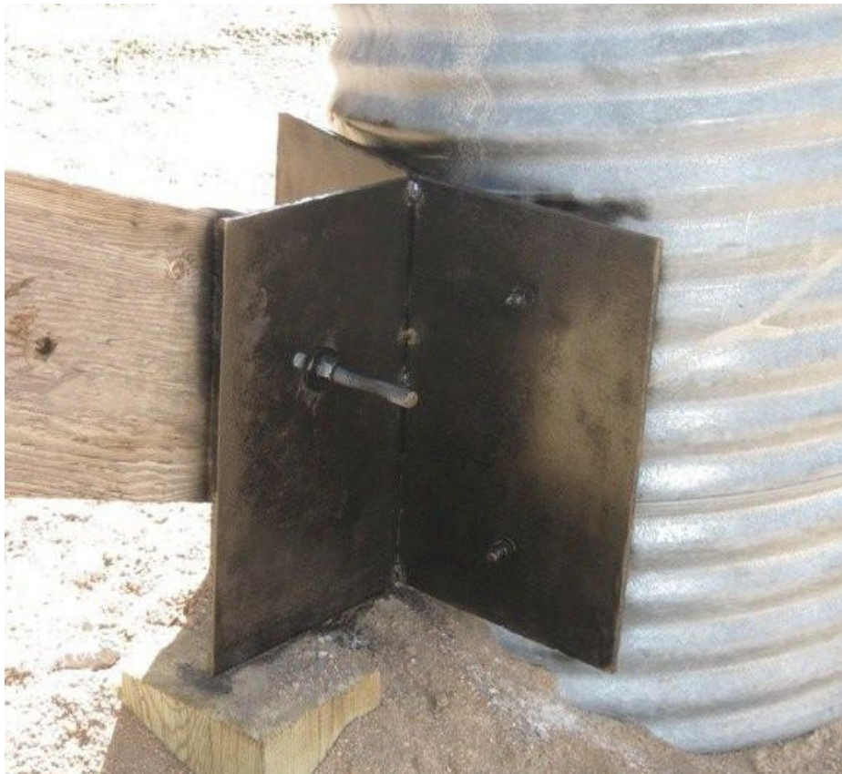
Fig. 16.12(G)-4 Photo of Timber Pile Repair and Bracing Connection
