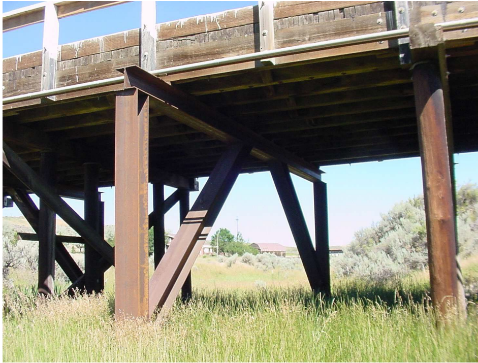
Fig. 16.12(H)-8 Photo of New Support Bent at Midspan
