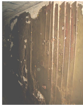
Fig. 16.12(L)-1 Sample Details for Repairing the concrete bottom slab of a box culvert
