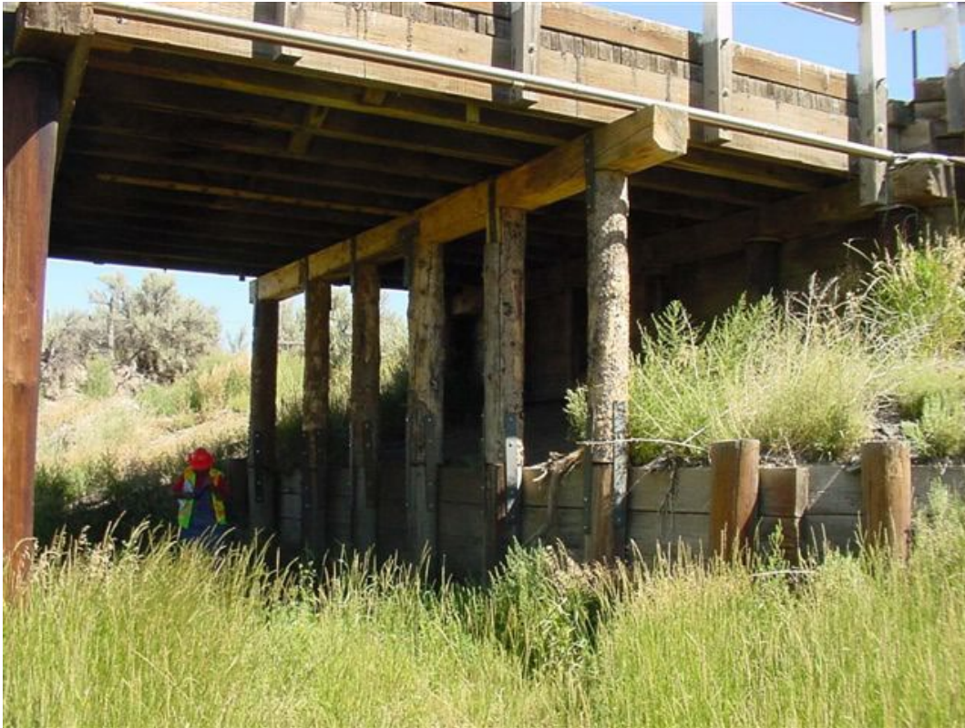
Fig. 16.12(H)-9 Photo of New Timber Bent
