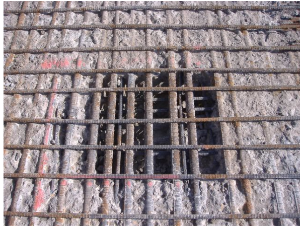
Fig. 16.12(C)-5 Close-up Photo of Deck Rehabilitation
