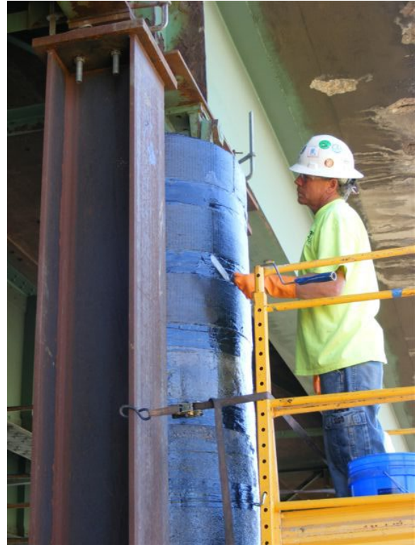
Fig. 16.12(D)-7 Photo of Fiber Wrap
