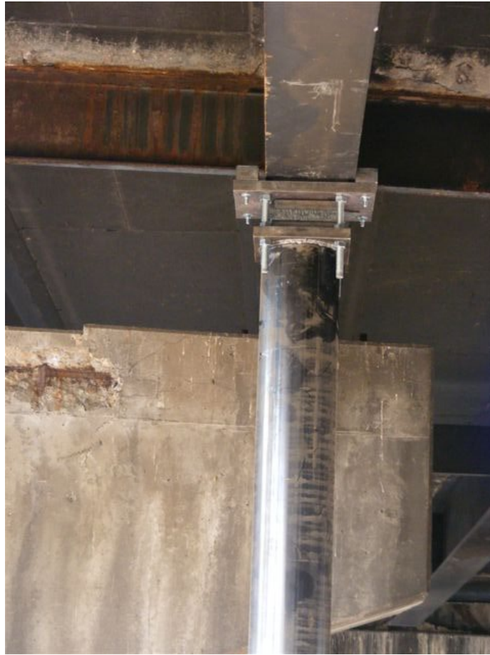
Fig. 16.12 (I)-3 Photo of Falsework to support a steel girder
